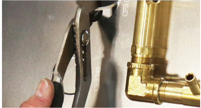
Photo 2: Breaking the Knockouts
