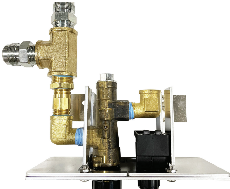
Photo 11b: Final Assembly Configuration
