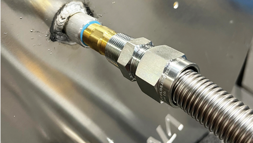
Photo 18: Connecting the Flex Line
