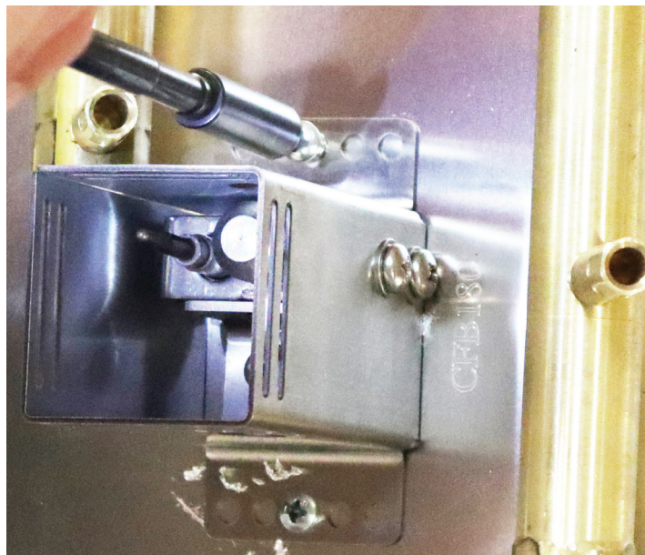
Photo 5: Securing the Pilot to the Plate/Pan
