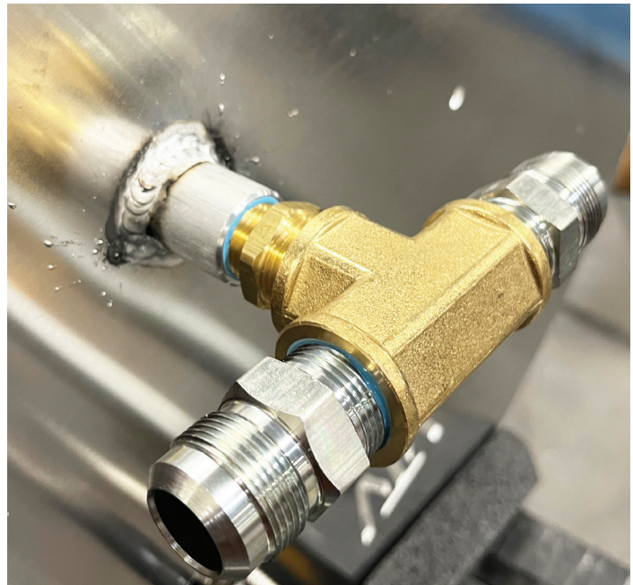
Photo 19b: Final Assembly Configuration
