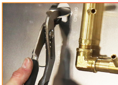
Photo 2: Breaking the Knockouts
