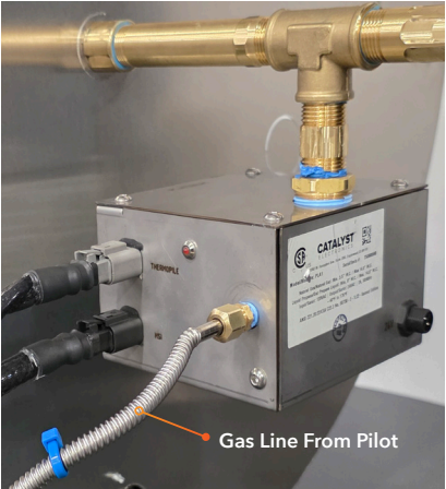
Photo 11: Connecting the Gas Line From the Pilot to the Valve
