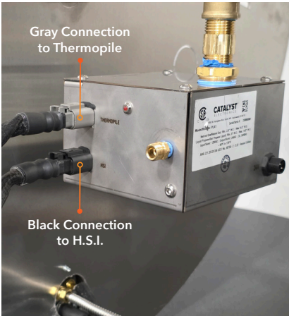
Photo 10: Electronic Connections from the Pilot to Valve
