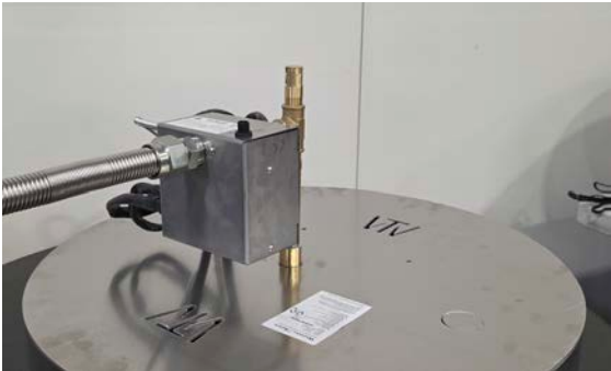
Photo 21: Attaching the Flex Line
