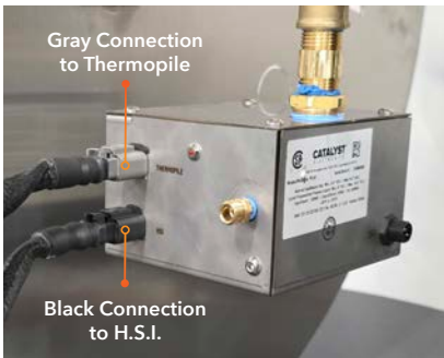
Photo 10: Electronic Connections from the Pilot to Valve
