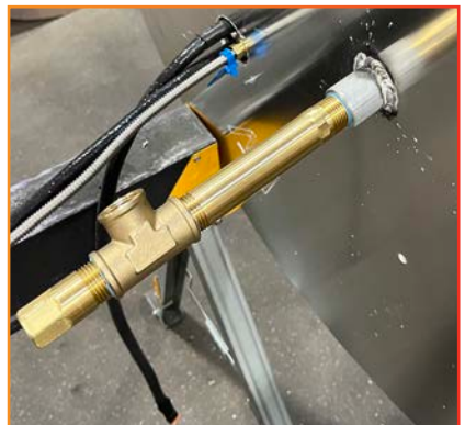
Photo 7b: Installing the Drip Leg
