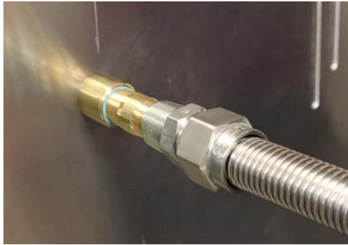
Photo 18: Connecting the Flex Line
