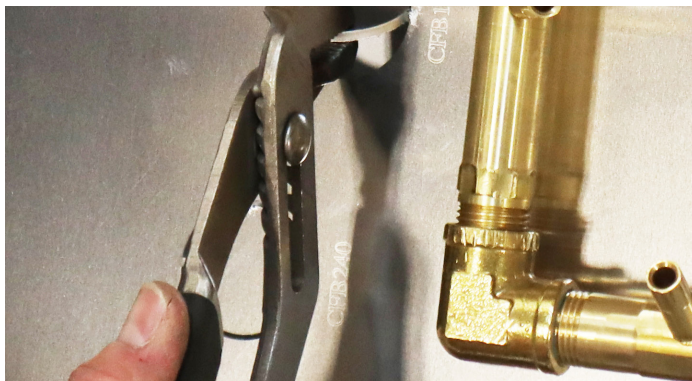
Photo 2: Breaking the Knockouts
