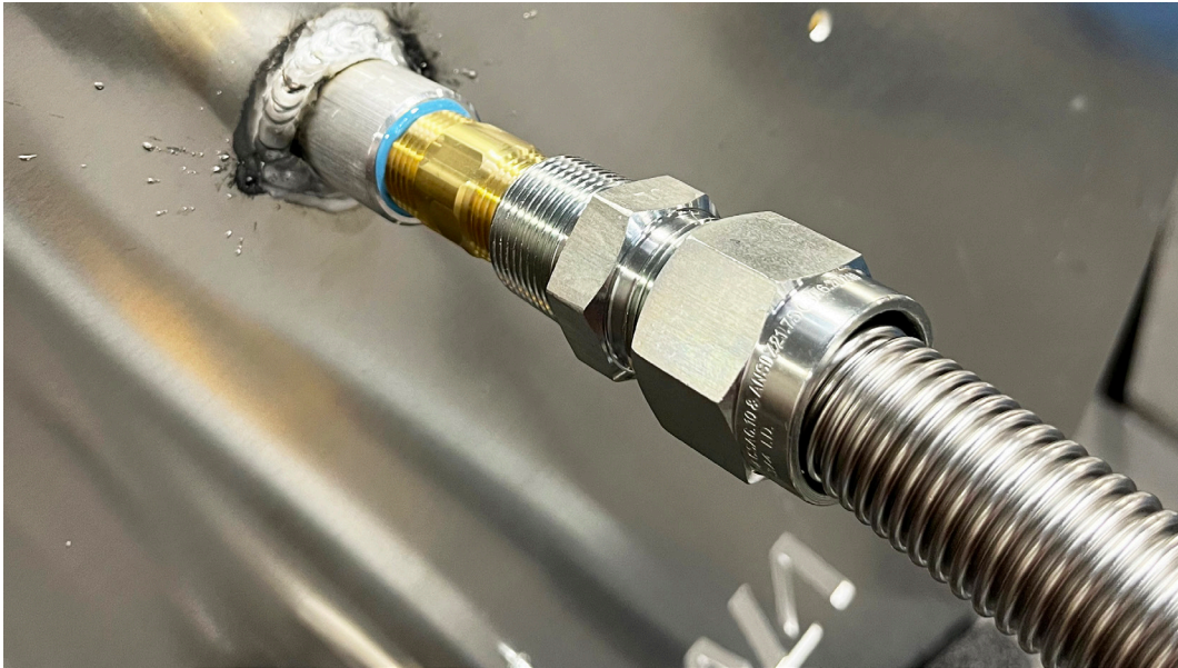
Photo 18: Connecting the Flex Line
